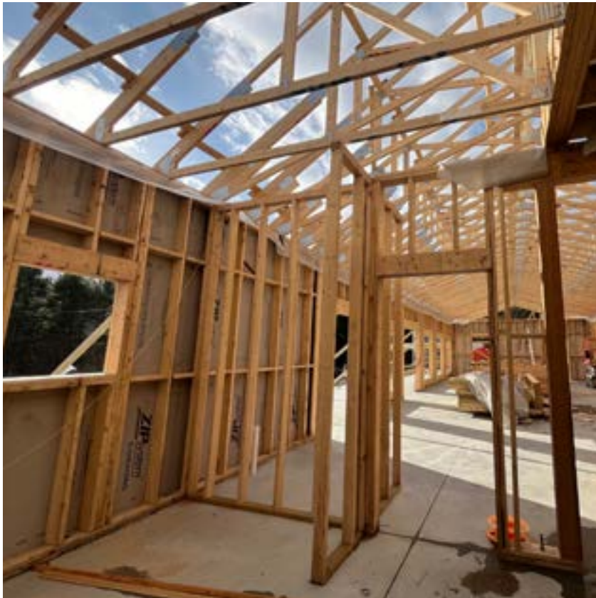
3. Framing is erected in what will be the state-of-the-art commercial kitchen.
